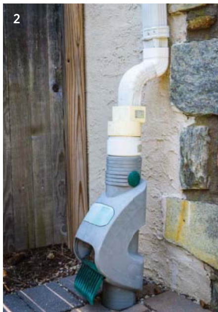
1. A water matrix module sits on top of permeable pavers. 2. A self-cleaning first flush rain filter removes dirt and debris from roof water. 3. Even without a pond, this water feature is attractive to wildlife. 4. An overflow pipe from the water storage area is directed into the rain garden. 5. A rain barrel can be capped with a mini green roof.
